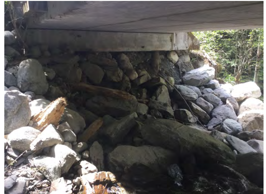
Left Bank Abutment when facing downstream
