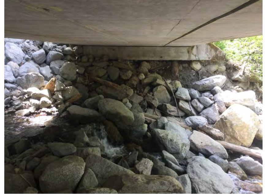
Left Bank Abutment when facing downstream
