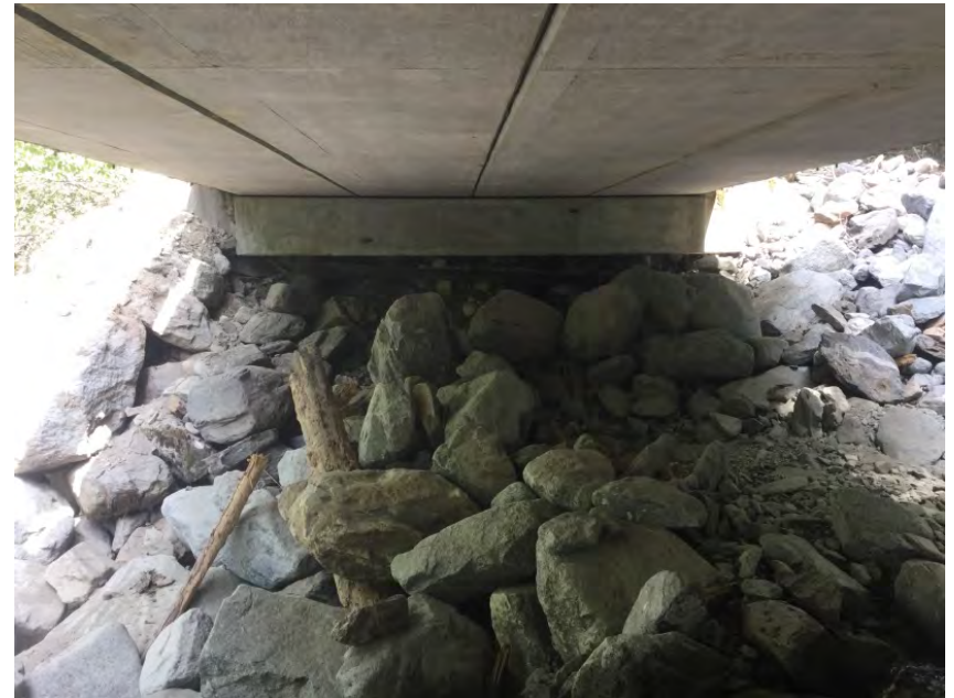
Right Bank Abutment when facing downstream
